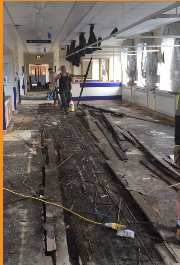
Removal of oak beams exposing bitumen.
